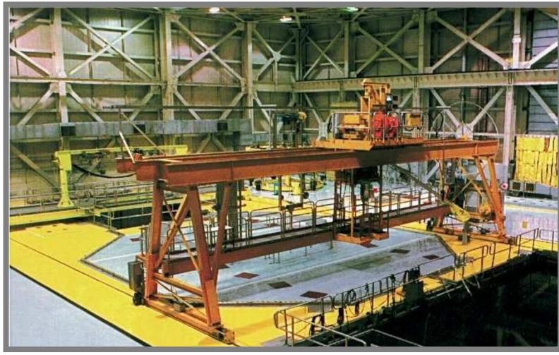
Lifting the Containment closure head
